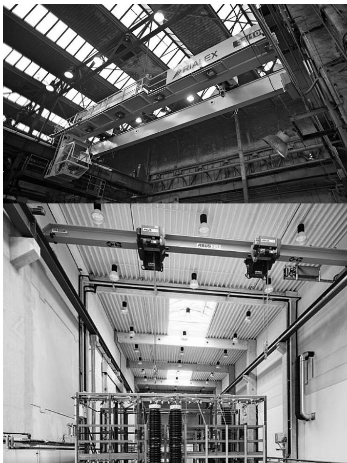
Fig. 1. Steel hall with the gantry ( http://www.zksgrzelak.eu/pl/belki-suwnicowe ).
