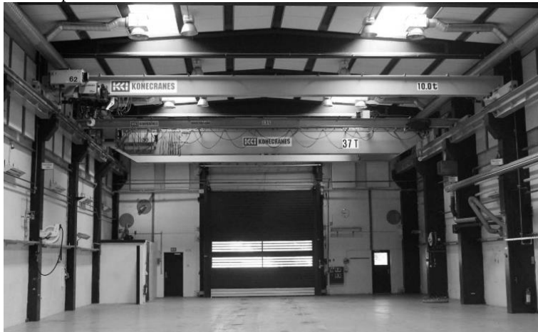
Fig. 2. Steel industrial hall with two gantry cranes ( http://www.ofertymaszyn.com/ ).
